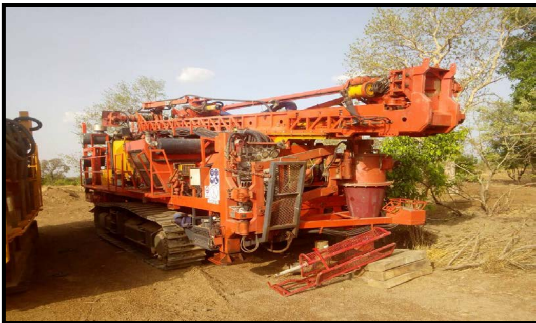
Figure 4: Drill Rigs on site at Gbane
