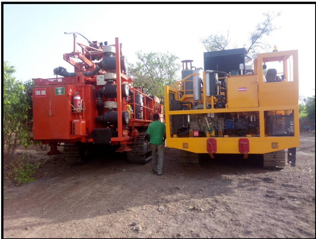
Figure 1: Geodrill rig and compressor on site at Gbane.
